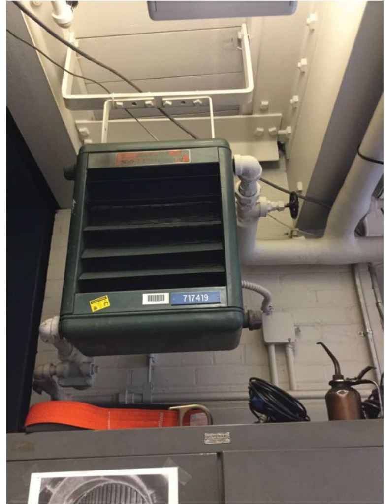
Equipment ID#: 717419 | Description: TERMINAL UNIT HEATER
